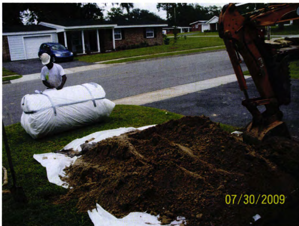
Picture 2: Containment of UST at 1414 Albatross after completion of work.
